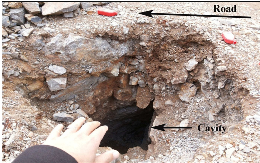
Figure- 1: Shows one of the cavities appears on the surface due to the cutting process.
